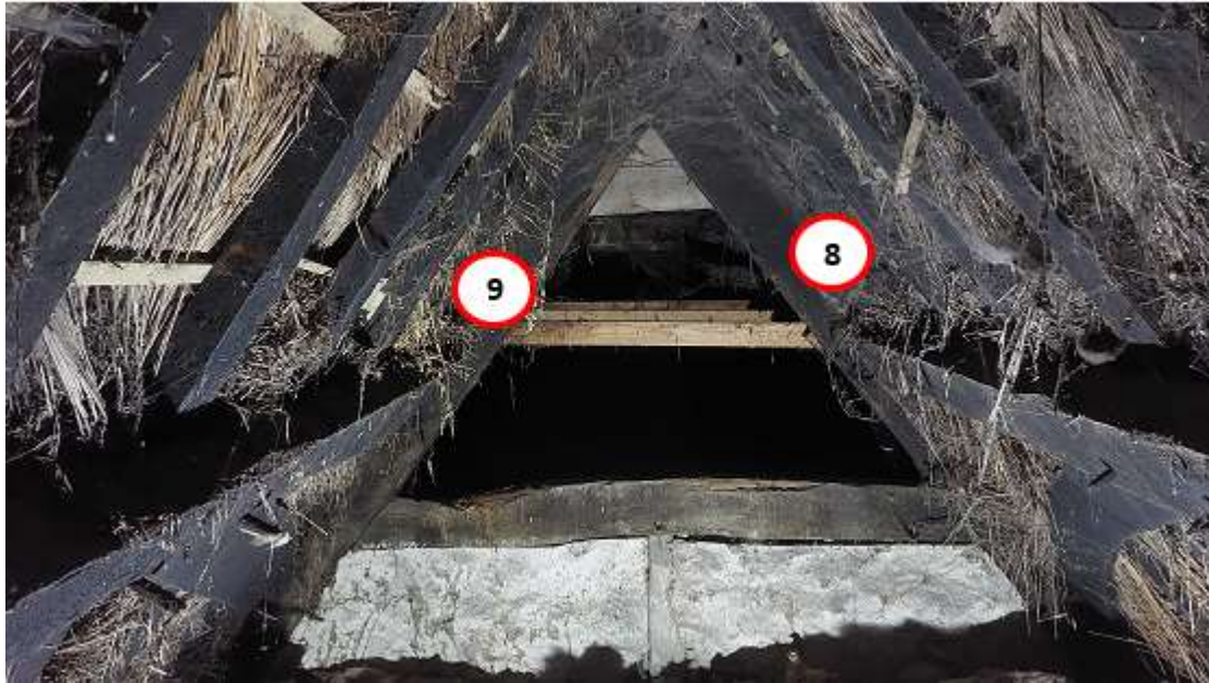
Figure 3c: Annotated photograph to show sampled timbers to truss 4 (viewed looking south) (see Table 1 and Figure 2)
