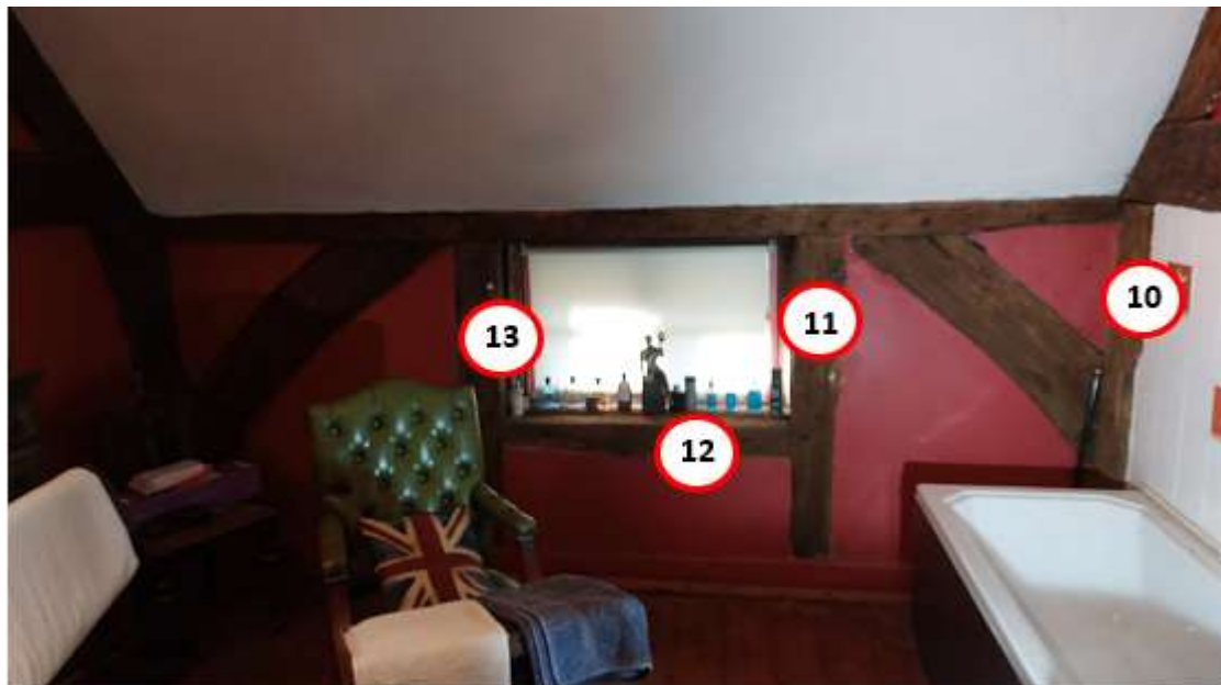
Figure 3d: Annotated photograph to show sampled timbers to bay 1 (from north) looking west (towards the road frontage) (see Table 1 and Figure 2)
