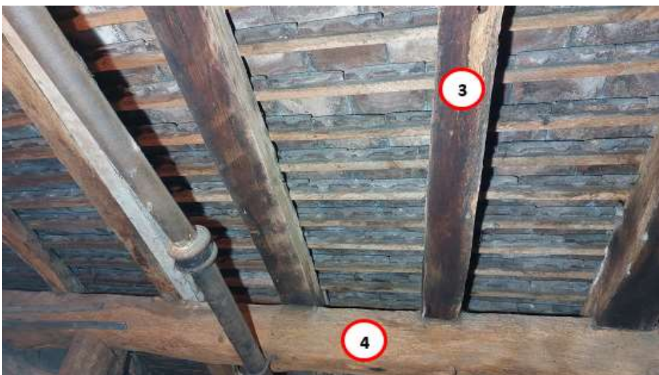
Figures 3a–c: Front range roof - annotated photographs to help identify sampled timbers (see table 1 and Figure 2)
