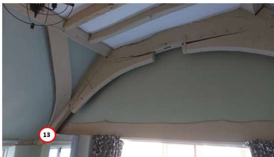
Figure 3f–h: First floor - annotated photographs to help identify sampled timbers (see table 1 and Figure 2)
