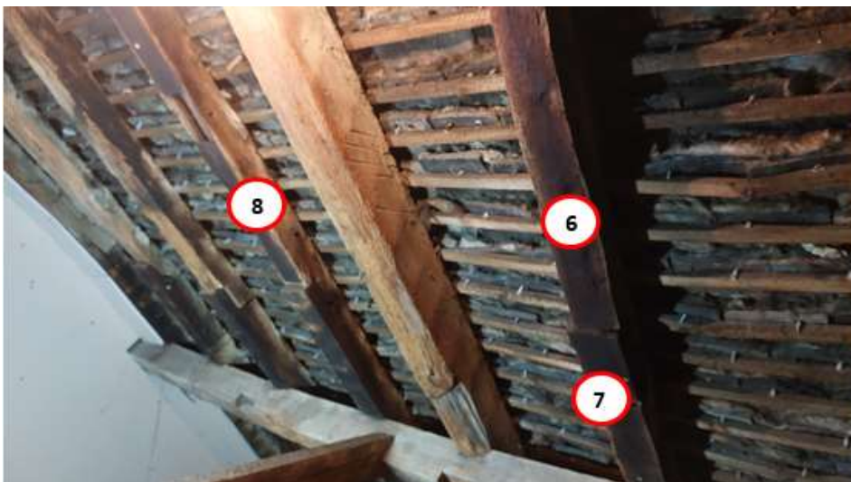
Figures 3d/e: Front range roof - annotated photographs to help identify sampled timbers (see table 1 and Figure 2)
