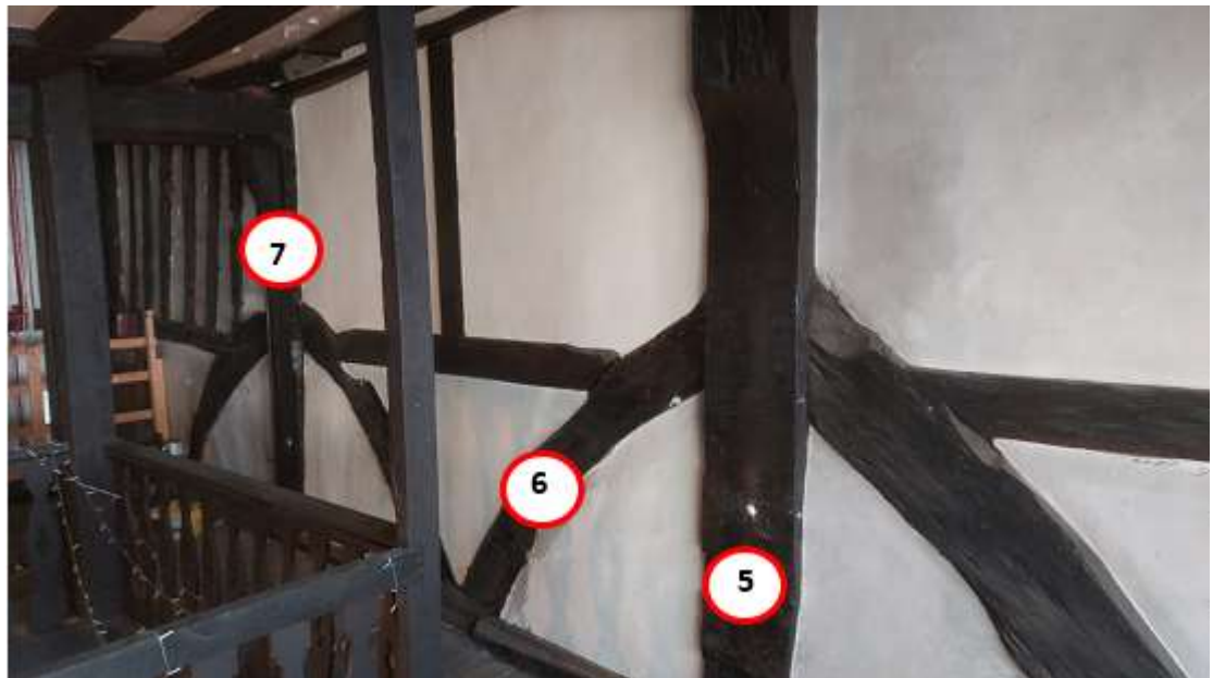
Figure 3b: Annotated photographs to help identify sampled timbers; truss 2, with truss 3 beyond, looking west (see Table 1 and Fig 2)
